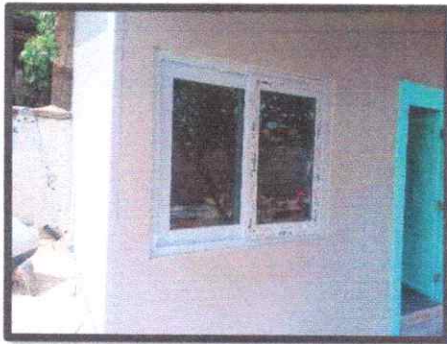
3.6.3.4 V4- Ventana PVC Termopanel – 1.64x1.14m
