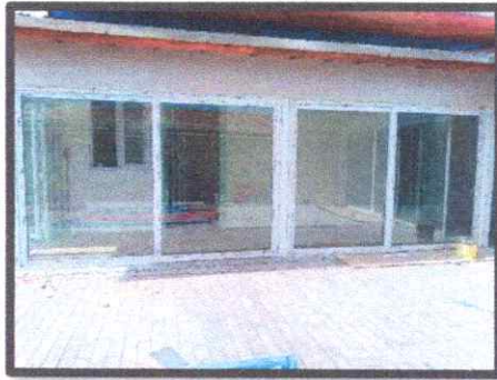
3.6.3.3 V3- Ventana PVC Termopanel – 1.12x1.40m
