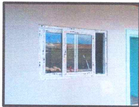
3.6.3.4 V4- Ventana PVC Termopanel – 1.64x1.14m
